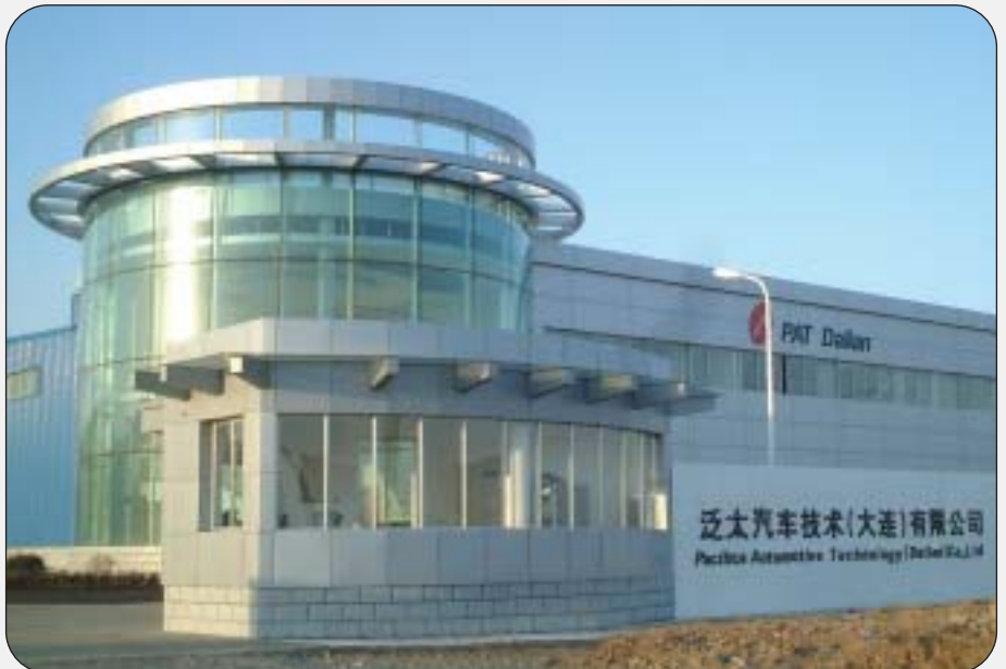
The new facility in Dalian, China, prepares for production
